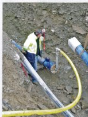
Figure 5: Inspection section end point
