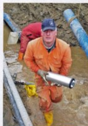
Figure 6: Pipe-Inspector after retrieval
