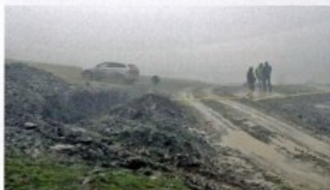
Figure 1: Site in over 2,000 m above sea level
